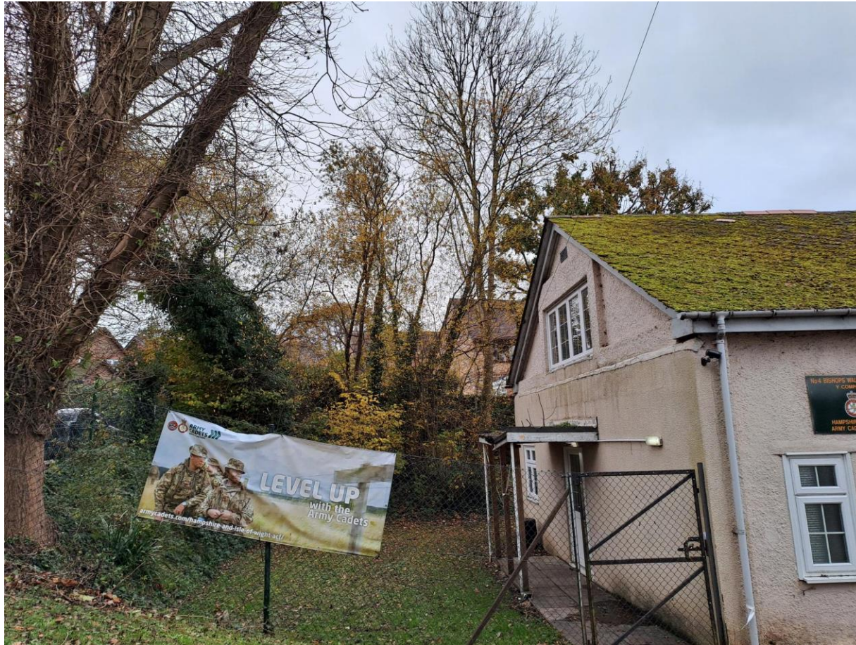
Photo towards northeast elevation
