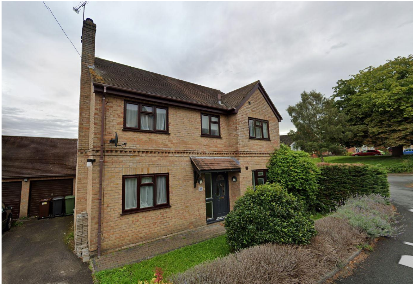
Street view towards southwest elevation
