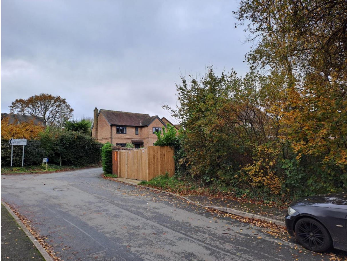
Photo towards northeast elevation
